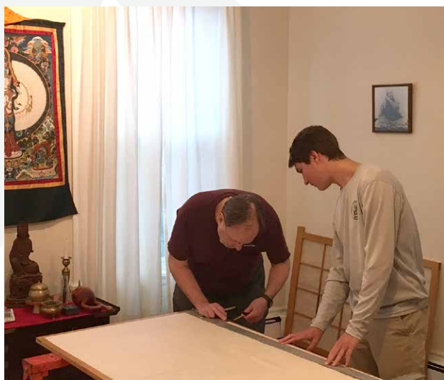
John O'Regan repairing the Dharma room rice paper door.
