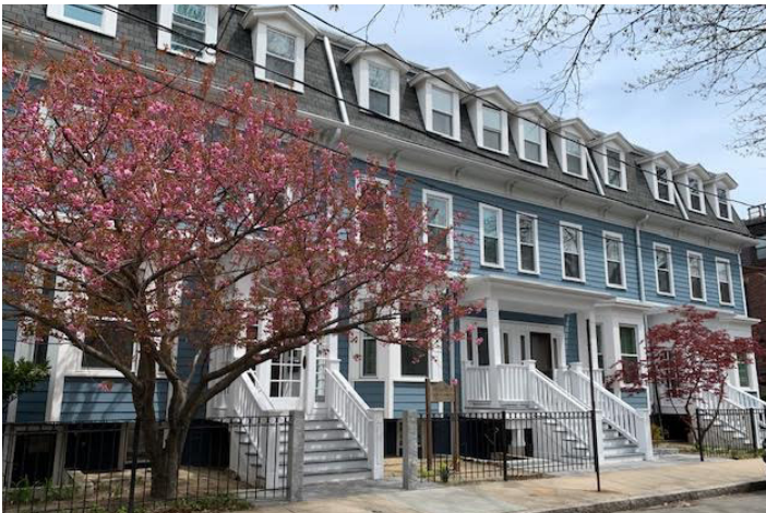
Completed Front Stairs Restoration Project
